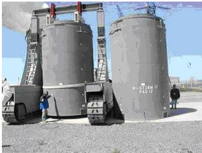
Dry casks removed from pool and reactor building en route to dry cask pad
